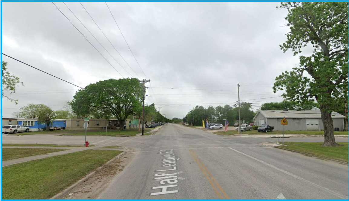
Photo 2.1 Half League Road with inlets and underground storm pipes
