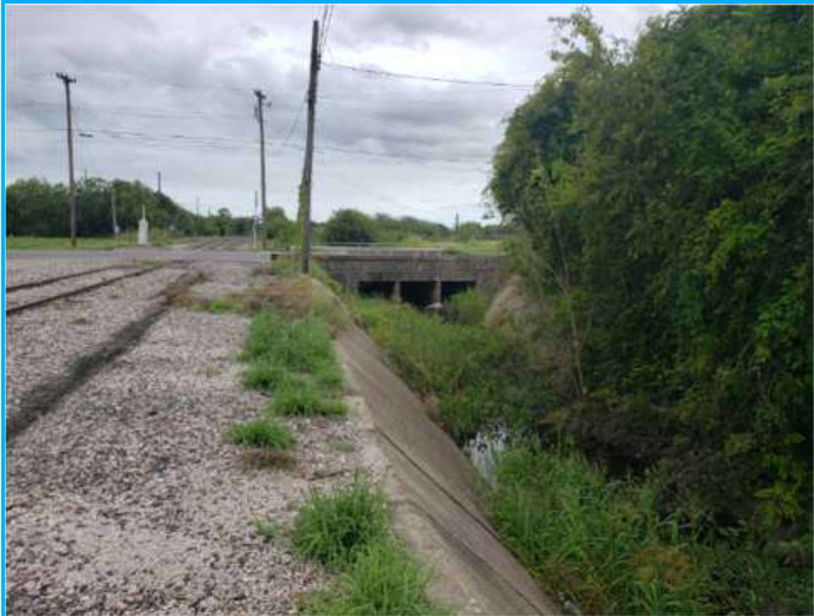
Photo 2.3 Section of Grassed Corporation Ditch
