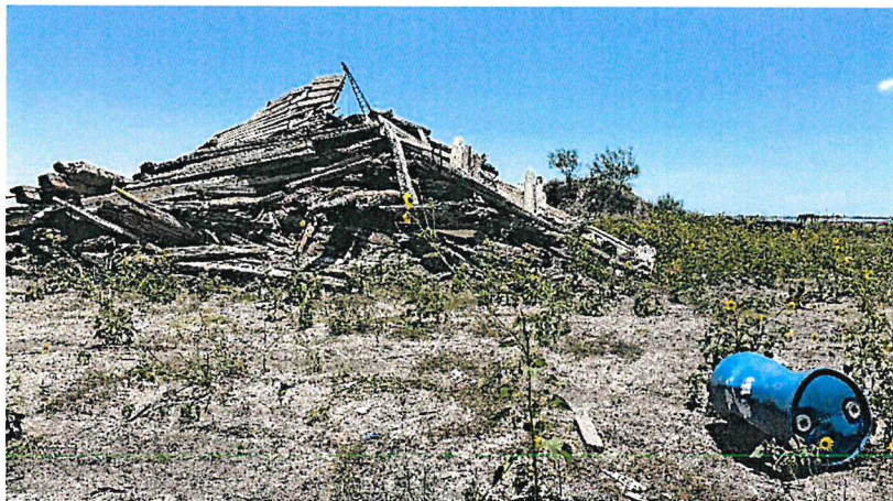
Looking generally east
