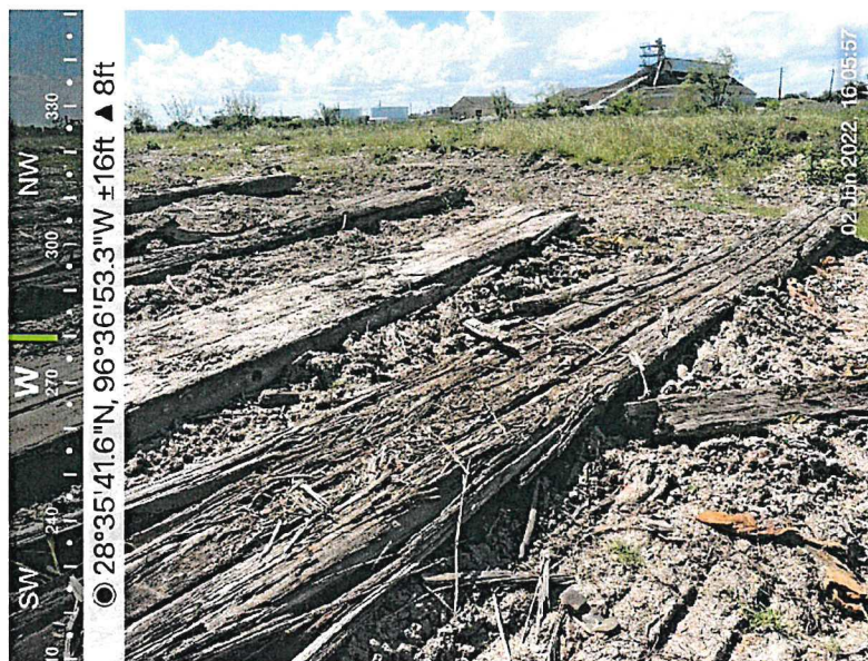
More wood equipment mats along the channel shore (looking generally northwest)
