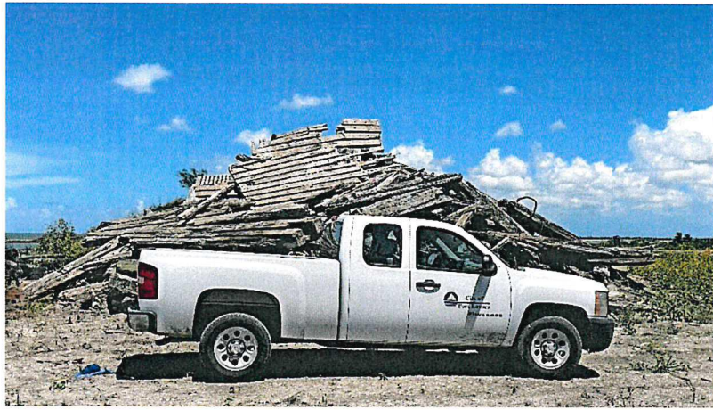
Generally looking south with truck in foreground for scale
