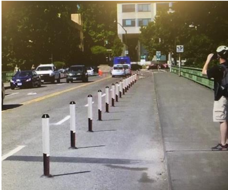
Reflectors Separating Pedestrians from vehicular traffic
